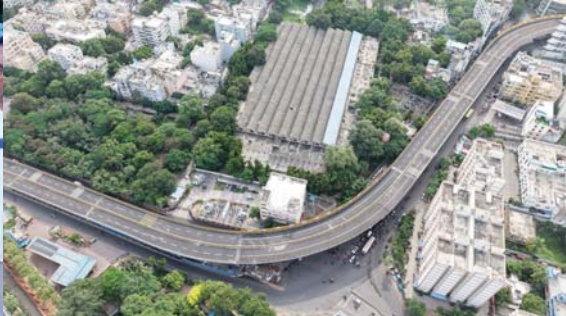
The four-lane Chanchalguda-Santoshnagar steel flyover, constructed at a cost of Rs. 620 crore, spans 3.2 km and is 16.6 metres wide.
